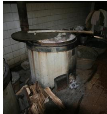
Wood fired boiler (Gidole hospital, Ethiopia)
