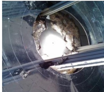
Iron block storage (NTNU)
