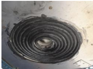
Oil pipe absorber (Durban)
