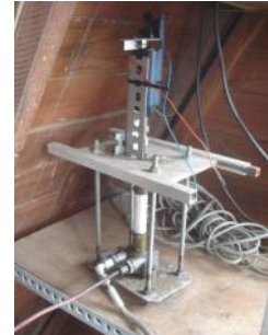
Motor and oil pump (Durban)
